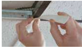
Applying GridMax Over T-bar Suspension Grid System
